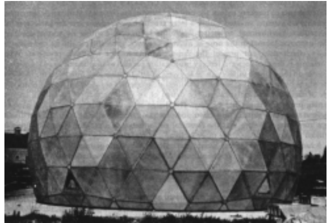
Figure R81 Rigid radome for ground-based antenna (from Skolnik, 1980, Fig. 7.29, p. 266, reprinted by permission of McGraw-Hill).
