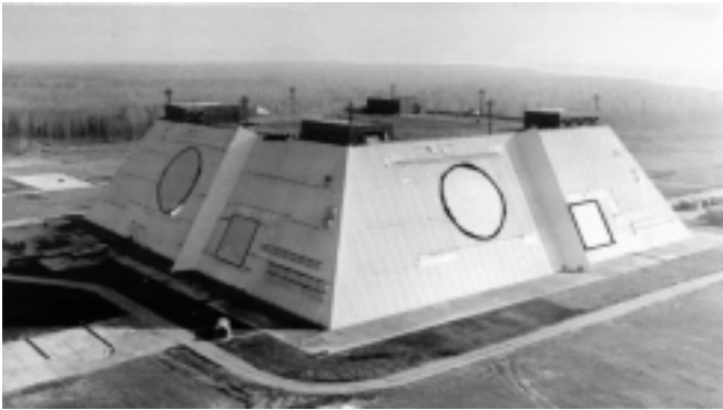
Figure R43 The Don radar, designed to support the Moscow ABM system and installed at Pushkino, northeast of the city.
