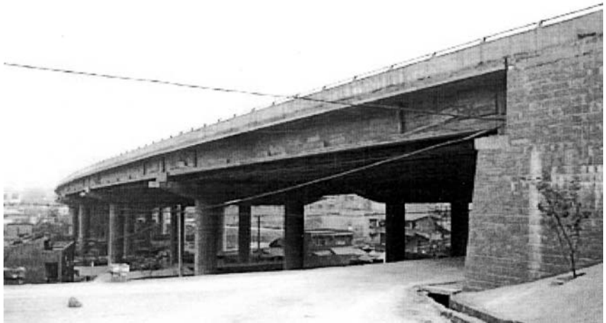
Figure 11 Photograph of the Hongcaofang crossroads concrete bridge in Chongqing, China.
