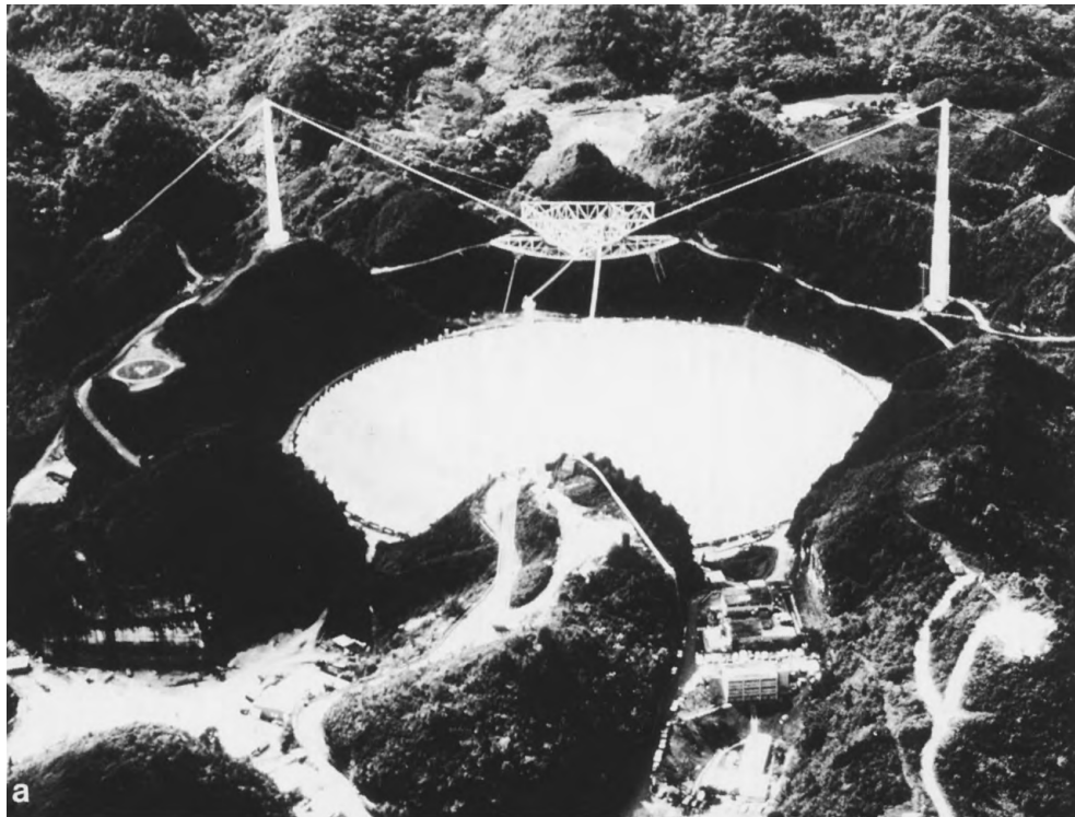
FIGURE 2 The Arecibo Observatory in Puerto Rico. (a) Aerial view prior to the recent upgrade. The diameter of the spherical reflector is 305 m. (b) A close-up view of the structure suspended above the reflector, showing the old 430-MHz line feed and the radome that encloses the new Gregorian secondary and tertiary subreflectors.
