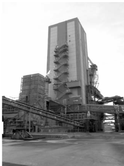
Lead battery recycling Recylex (Germany) (b)
