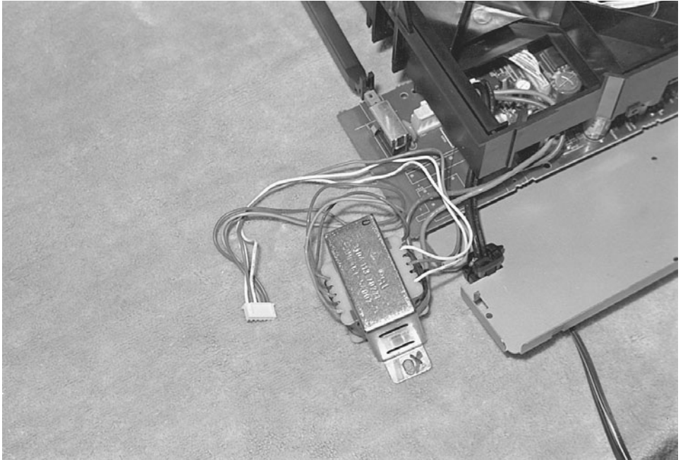
8-24 The shorted ac power transformer within a Magnavox CD changer.
