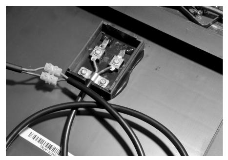
FIGURE 2-7: CONNECTING THE SOLAR PANEL
