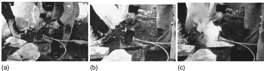
FIGURE 10.230 Exothermic bonding is the preferred method of joining the elements of a ground system. This photo sequence illustrates the procedure: (a) the powdered copper oxide and aluminum compound are added to the mold after the conductors have been mechanically joined; (b) final preparation of the bond before igniting; (c) the chemical reaction that bonds the materials together.
