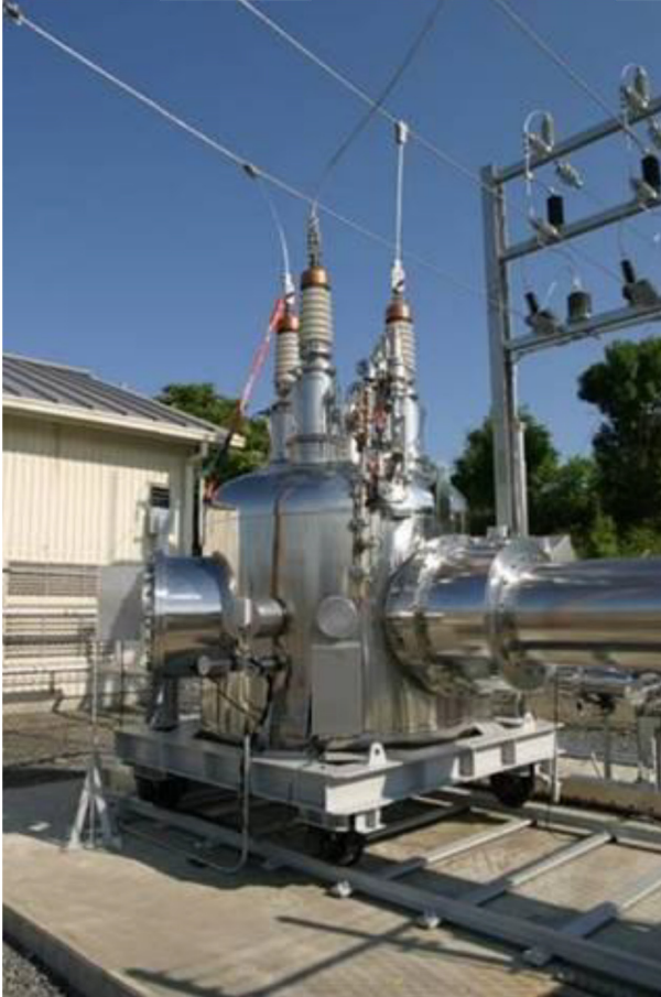
Figure 5.15 Three-phase termination/bushing used in the Albany project (Masuda et al., 2007). The termination skid is on rollers to accommodate the thermal contraction of the HTS core when it cools down.
