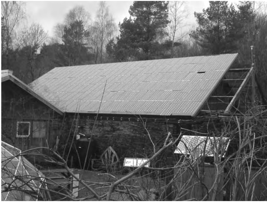
Figure 10-37 The 11 kW solar array at the Centre for Alternative Technology, U.K.
