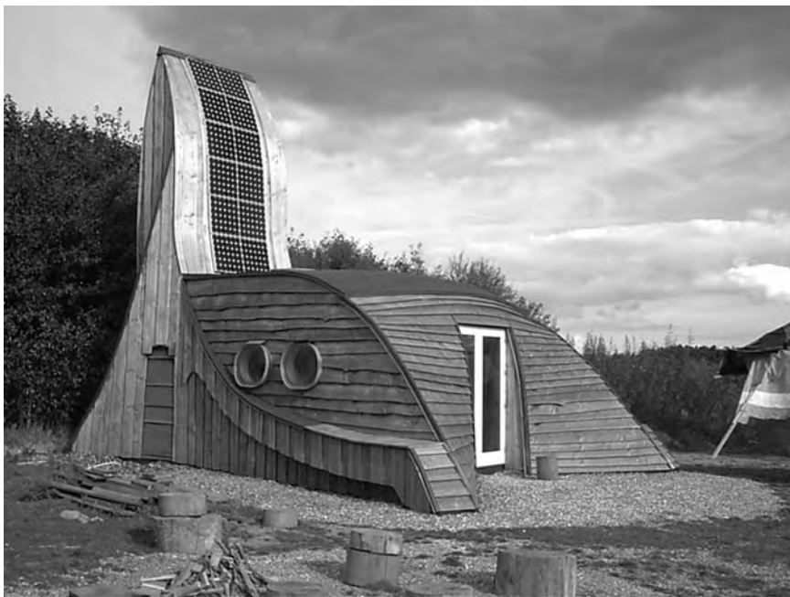
Figure 10-38 Photovoltaic cells creatively integrated into a building fabric. Image courtesy Jason Hawkes.
