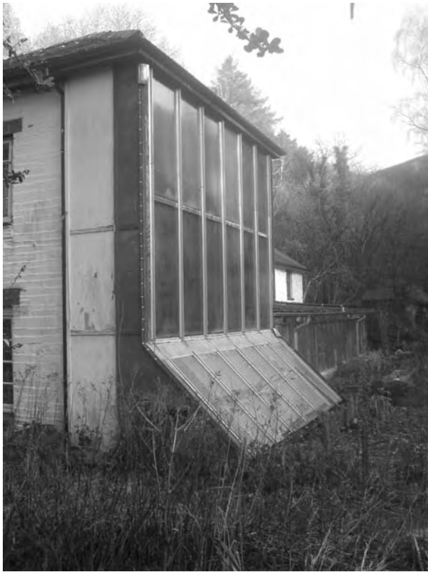
Figure 5-1 Trombe wall at CAT, U.K.
