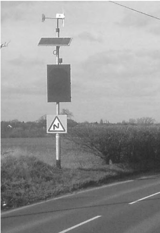
Figure 10-36 A road sign powered by renewable energy.
