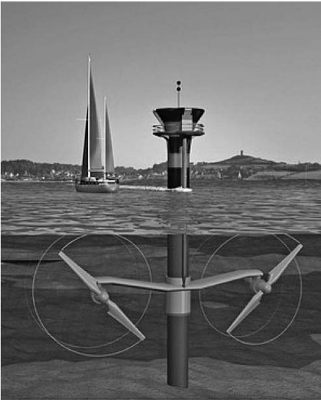
**FIGURE 13.9** A marine current tidal power-generating tower. (With permission from Marine Currents Turbine Ltd., Bristol, UK.)
