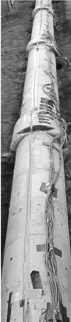
14.2 Reinforced concrete gravity pipeline with bell-and-spigot joint.
