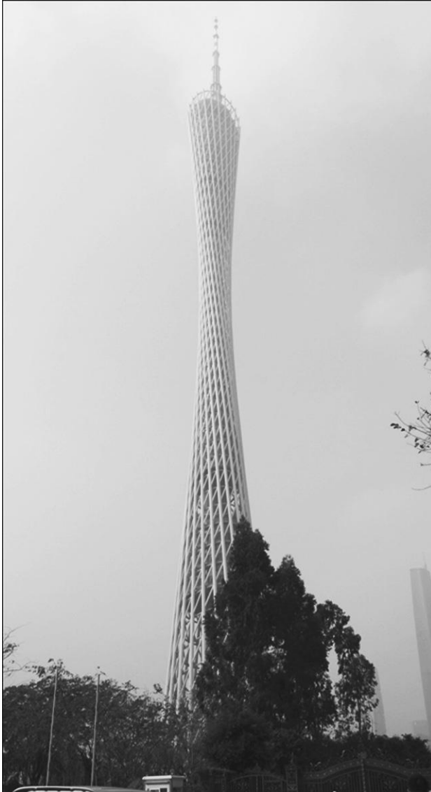
9.1 The Canton Tower (CT).
