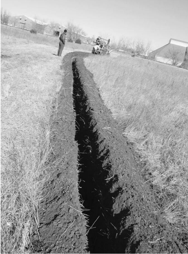
13.9 Digging of a trench to install the distributed sensing cable. (Source: Photo courtesy of SMARTEC.)
