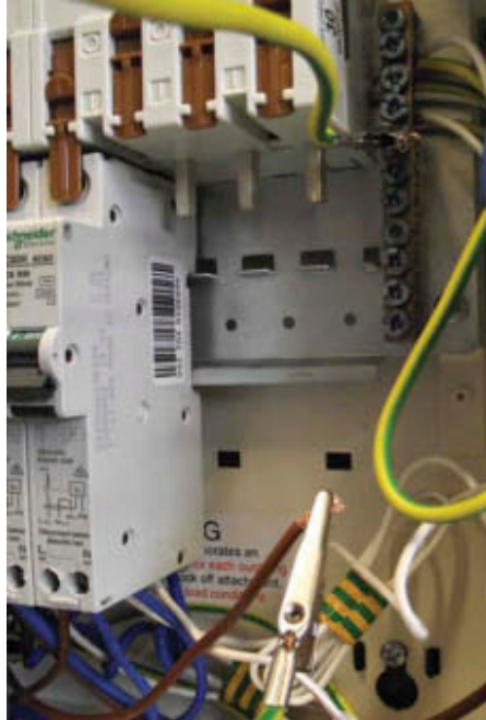
Figure 4.61 Line and earth terminal linked
