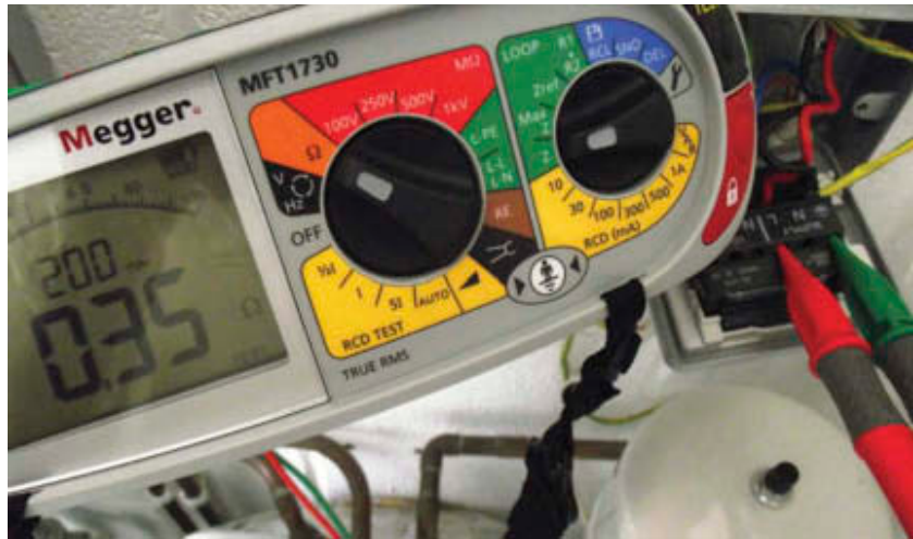
Figure 4.26 Probes on line and earth
