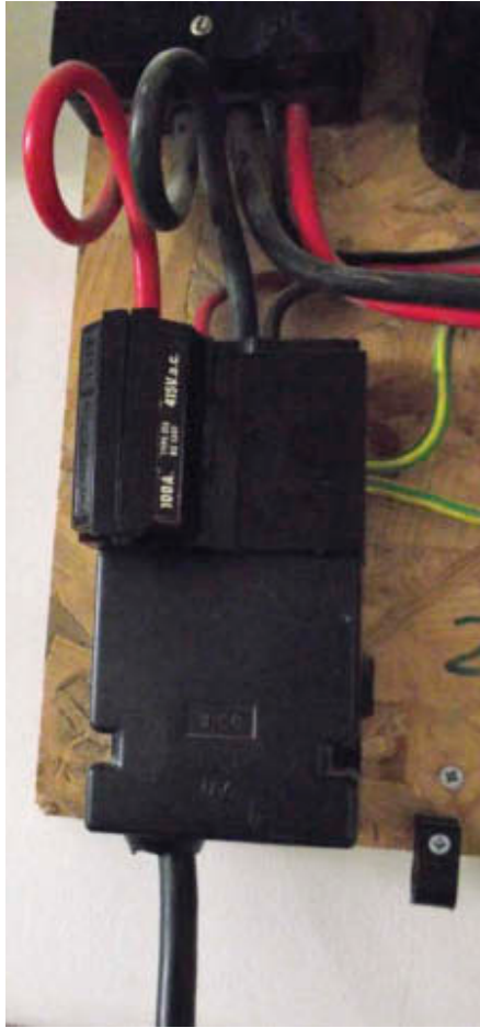
Figure 5.8 TN-C-S service head
