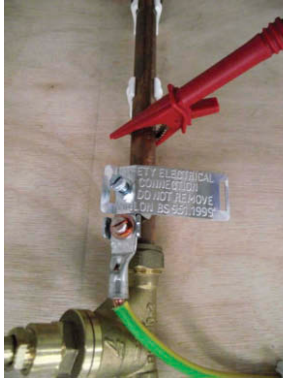
Figure 4.16 Second lead connected
