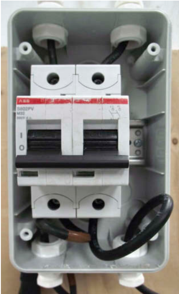
Figure 10.12 D.C. isolated
