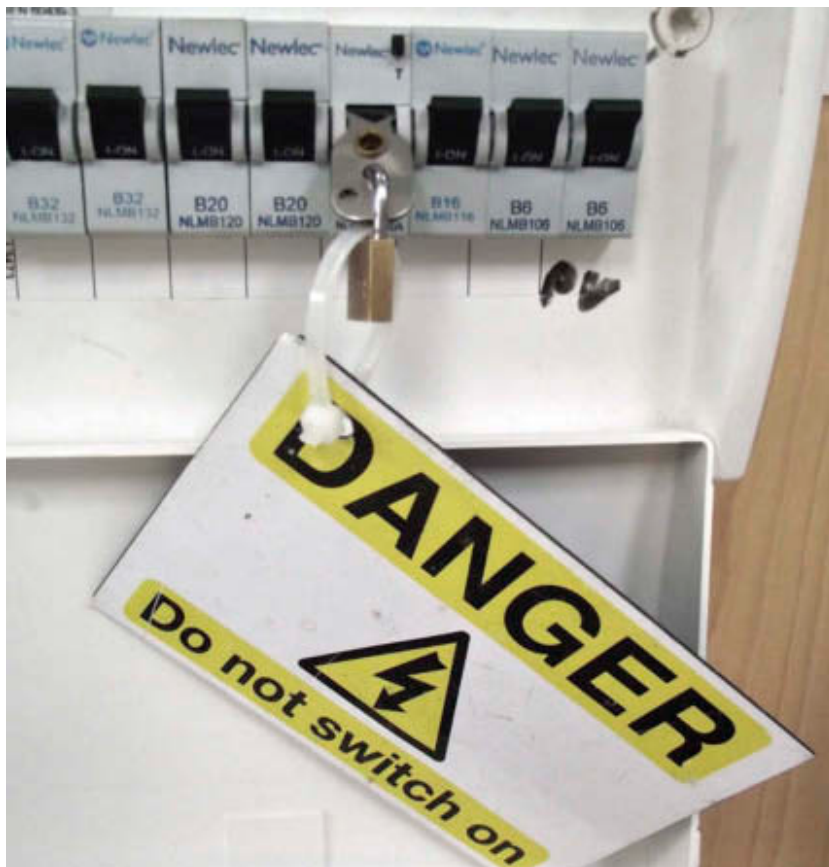
Figure 4.8 Locked off
