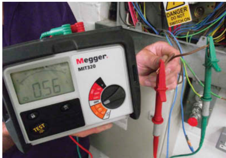
Figure 4.33 Test each end of the line conductor
