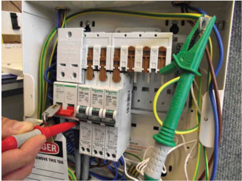
Figure 5.3 Tester connected
