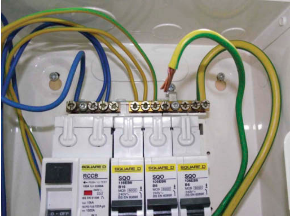
Figure 4.13 Bonding disconnected
