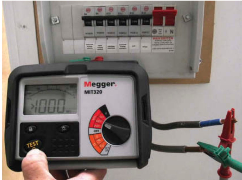
Figure 4.46 Test between live conductors
