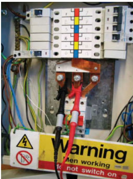
Figure 4.51c Test L1 to L2
