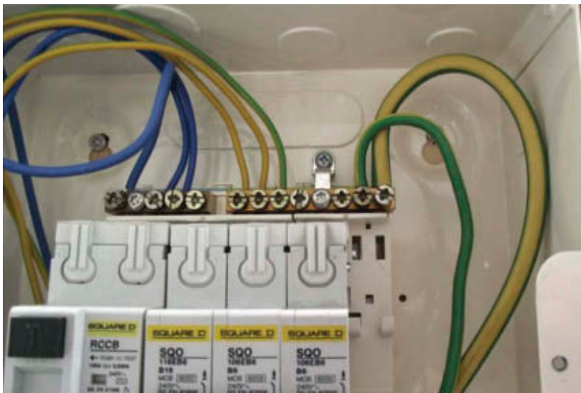
Figure 4.18 Reconnect bonding
