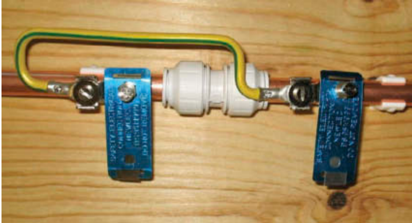
Figure 4.23 Fitting bonded across
