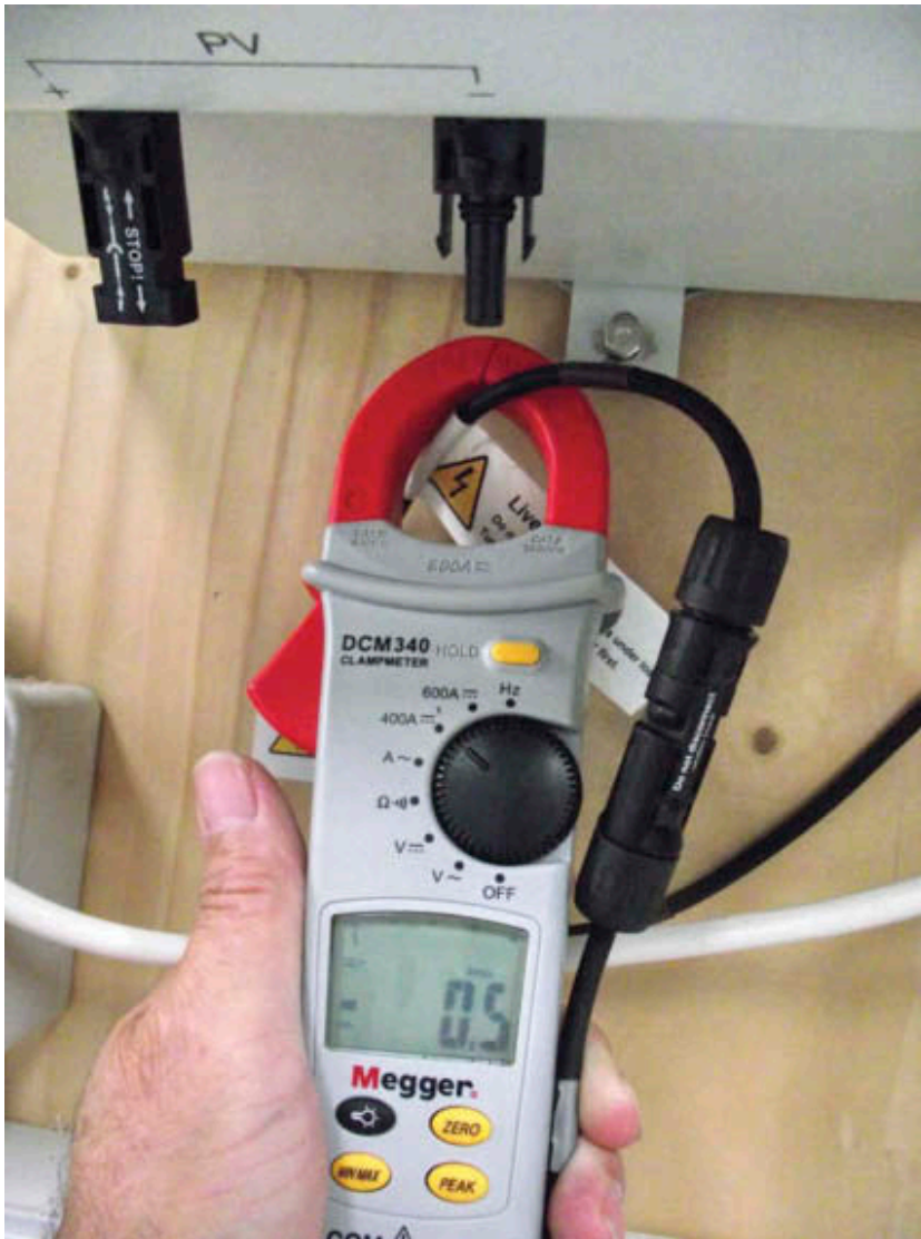
Figure 10.10 Current measurement using clamp meter
