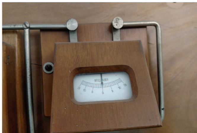
Figure 2.5 The differential voltage can be displayed on an old-style meter movement. Notice that this meter can swing to the left or right, depending on the current direction.
