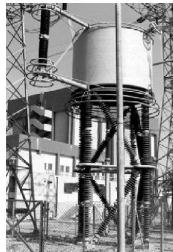
FIGURE 31.8 Installation of an air-cooled smoothing reactor.
