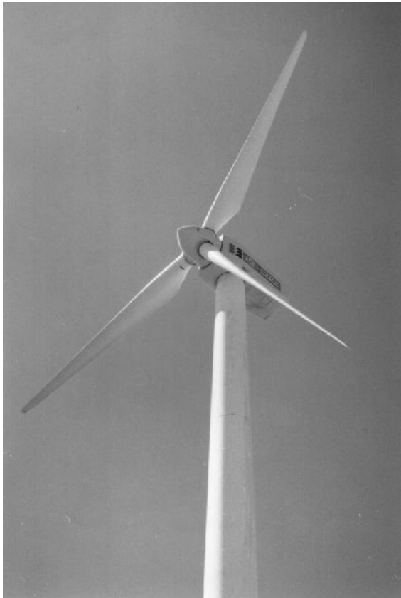
FIGURE 30.2 Wind turbine in Monteahumada (Spain). Made S.A. AE-41PV.
