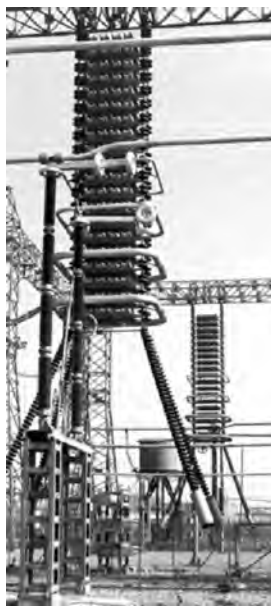
FIGURE 30.7 Installation of an ac filter in the switchyard.
