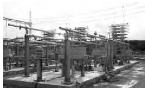
FIGURE 30.28 Installation of the triple-tuned filter at the Gurun station in Malaysia.
