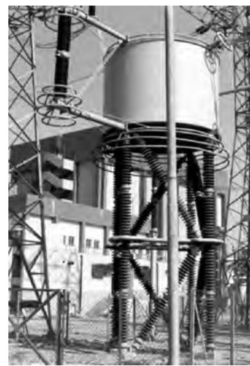
FIGURE 30.8 Installation of an air-cooled smoothing reactor.
