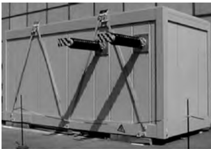
FIGURE 30.27 Compact outdoor container with an active dc filter.
