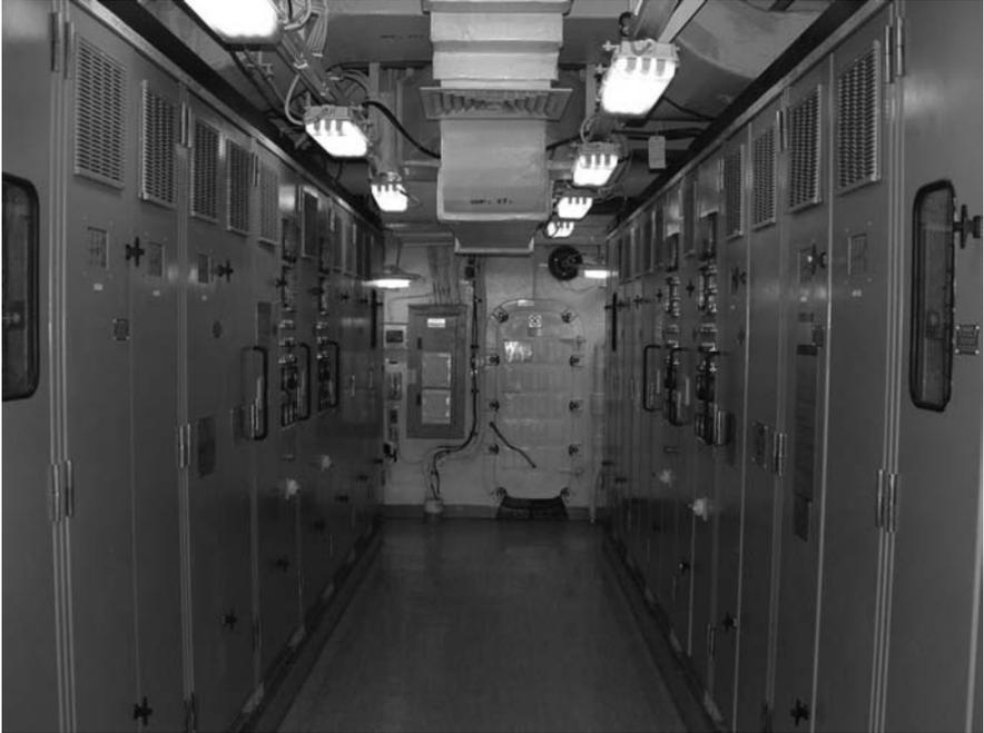
Figure 15.7 Two medium-voltage cycloconverter propulsion drives onboard a ship
