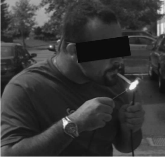
Figure 2.6 Dangerous dc arc-fault (do not try this at home)
