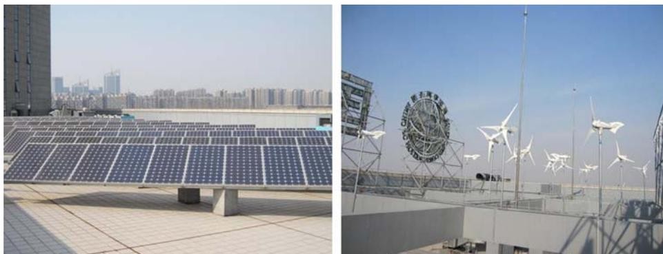
**Figure 6.67** Wind/PV microgrid system at the Nanjing Power Supply Company [13]
