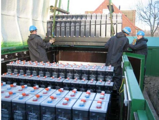
**Figure 6.23** Installation of the batteries
