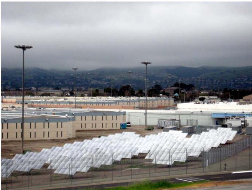
**Figure 6.29** Recent photo of Santa Rita Jail, with ground mounted tracking solar PV in the foreground and batteries and fuel cell directly behind
