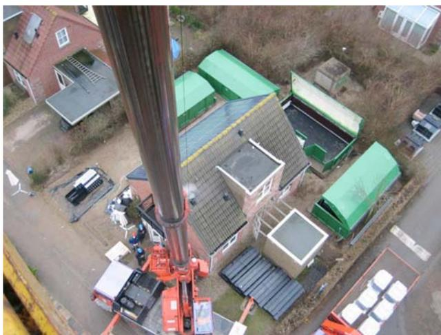
**Figure 6.22** View of the cottage and the battery containers. The distribution transformer is in the concrete box at the top right of the open container
