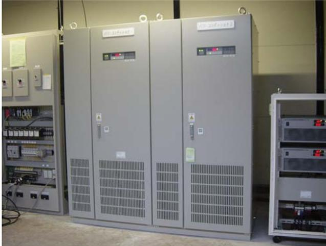
**Figure 6.51** PV inverter to compensate for imbalances between the three phases
