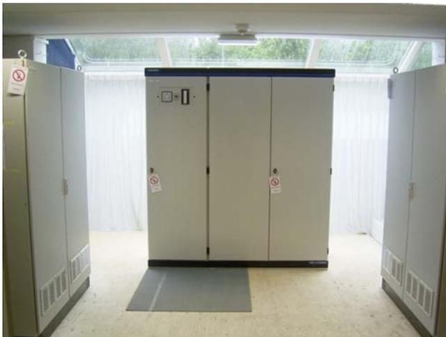
**Figure 6.21** The system room with switchgear cabinet (center) and inverters
