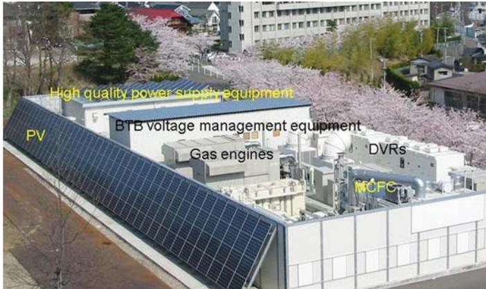
**Figure 6.54** Sendai project's compensating equipment and generators
