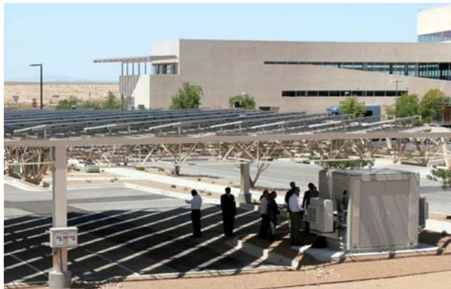
**Figure 6.40** Solar PV array at the Aperture Center microgrid
