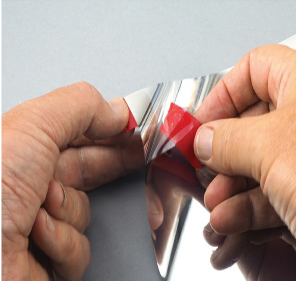
Figure 3-14: Removing the plastic backing from the reflective window film
