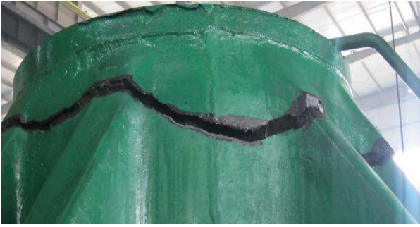
Fig. 1 Fracture of cubic hinge sleeve in the bottom
