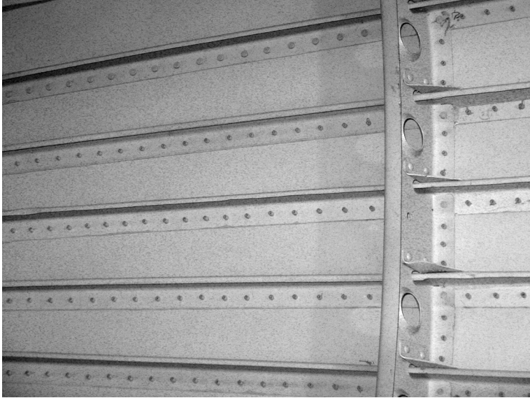
9.1 Example of a typical aeronautical structure, composed of a riveted stiffened skin.
