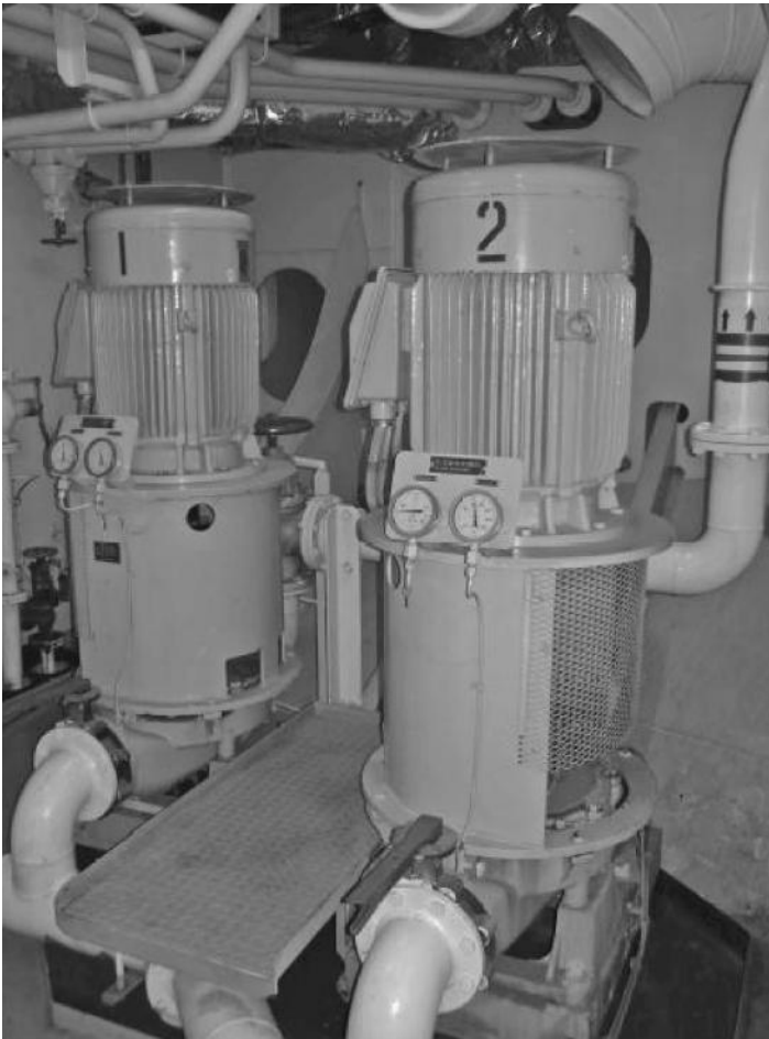
FIGURE 4.2 Vertical shaft motor saves footprints in ships and in city centers. (Courtesy of Raul Osigian, U.S. Merchant Marine Academy.)
