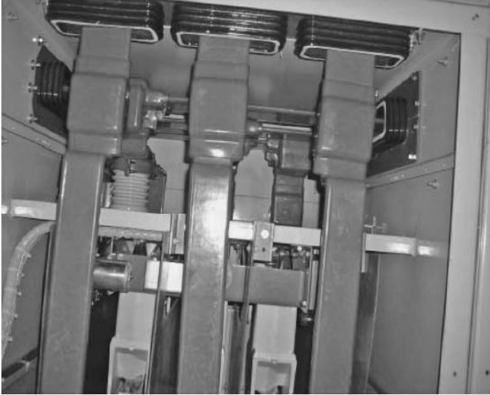
FIGURE 7.9 High-voltage bus bars in switchgear through porcelain bus ducts: cast epoxy insulated with joints covered by removable boots. (From Myers Power Products, Inc. With permission.)
