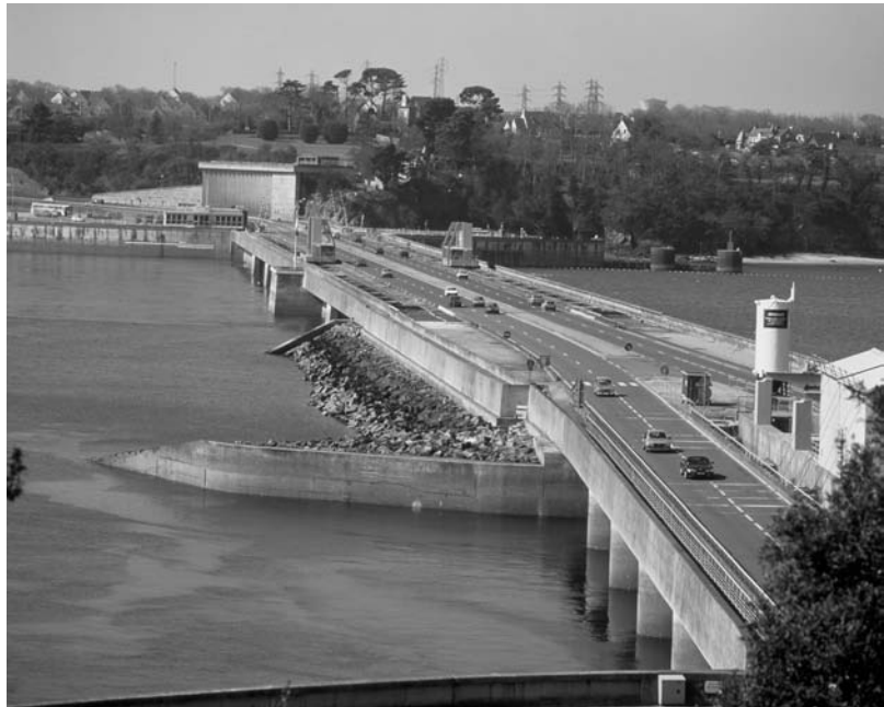
Fig. 37.18 A ‘dam’ built across the mouth of an estuary harnesses the potential energy of the tides
