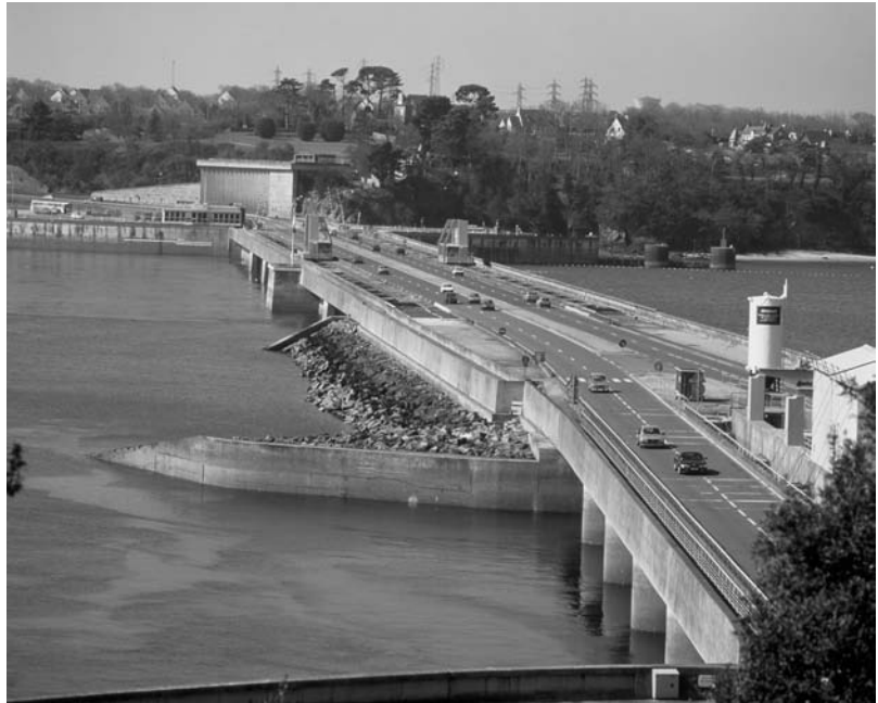
Fig. 39.18 A ‘dam’ built across the mouth of an estuary harnesses the potential energy of the tides
