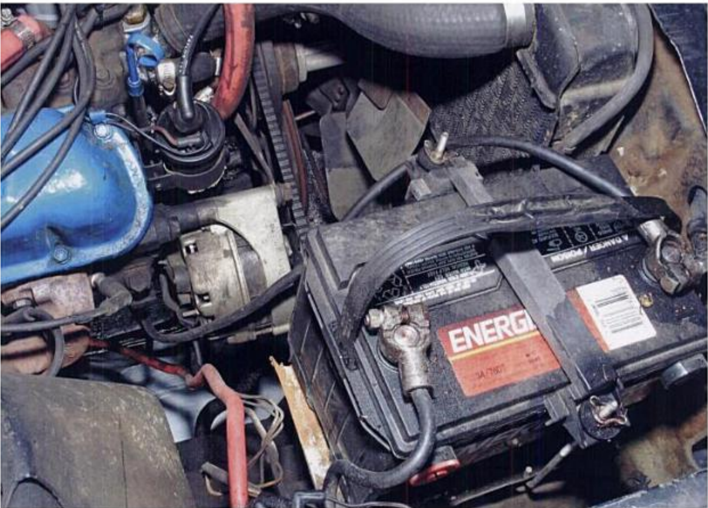
Two power sources found in all vehicles—the storage battery and alternator (or generator in older vehicles).
