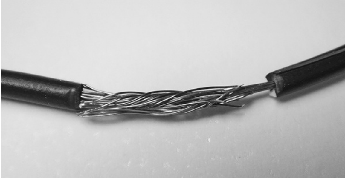
FIGURE 6-16 Stranded wires twisted together.
