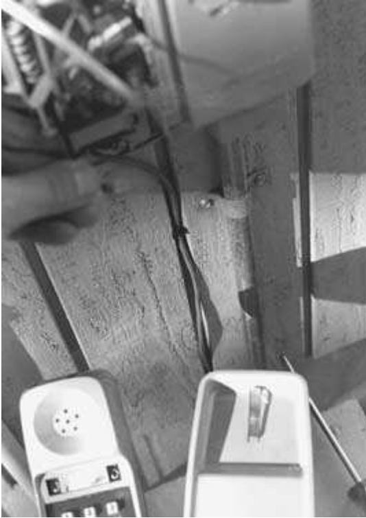
FIGURE 8-7 Unplug the test phone and reconnect the modular plug into the interface jack.
