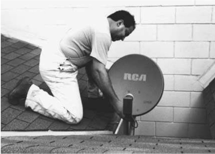
FIGURE 6-7 A roof-mounted DBS dish being installed and adjusted.
