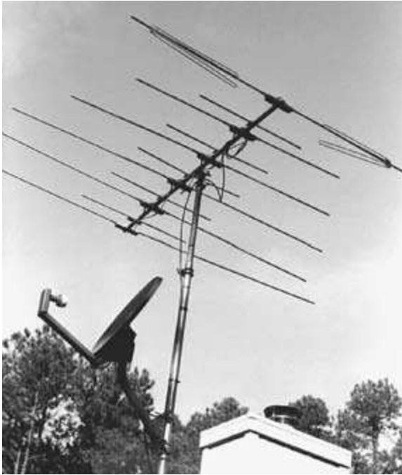
FIGURE 6-1 The satellite dish is shown mounted on a mast below a conventional TV antenna .
