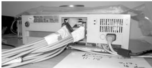
Figure 8-16. ISA card cable bundles
