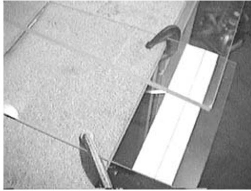
Figure 2-52. Remove excess material
