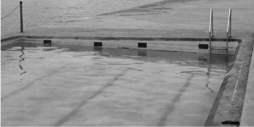
Figure A1.5.1. Swimming pool with an apparently sloping water surface.
