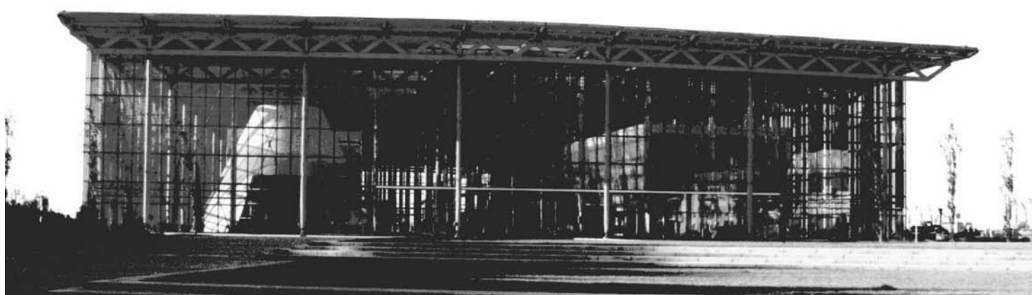
Figure C4.4.19. The Mont Cenis Academy at Herne-Sodingen.
