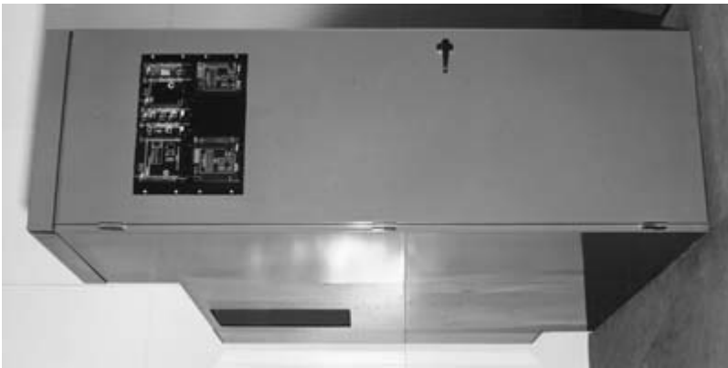
Fig. 14.7 (a) A modern 12 kV vacuum circuit-breaker equipment ( left & centre ). (b) A modern 'ring main unit' equipment using SF 6 technology ( right ).
