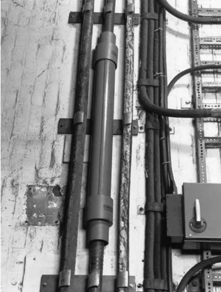
Fig. 19.9 Typical profile of modern straight through joint in 11kV polymeric-insulated cables ( Pirelli Cables Ltd ).
