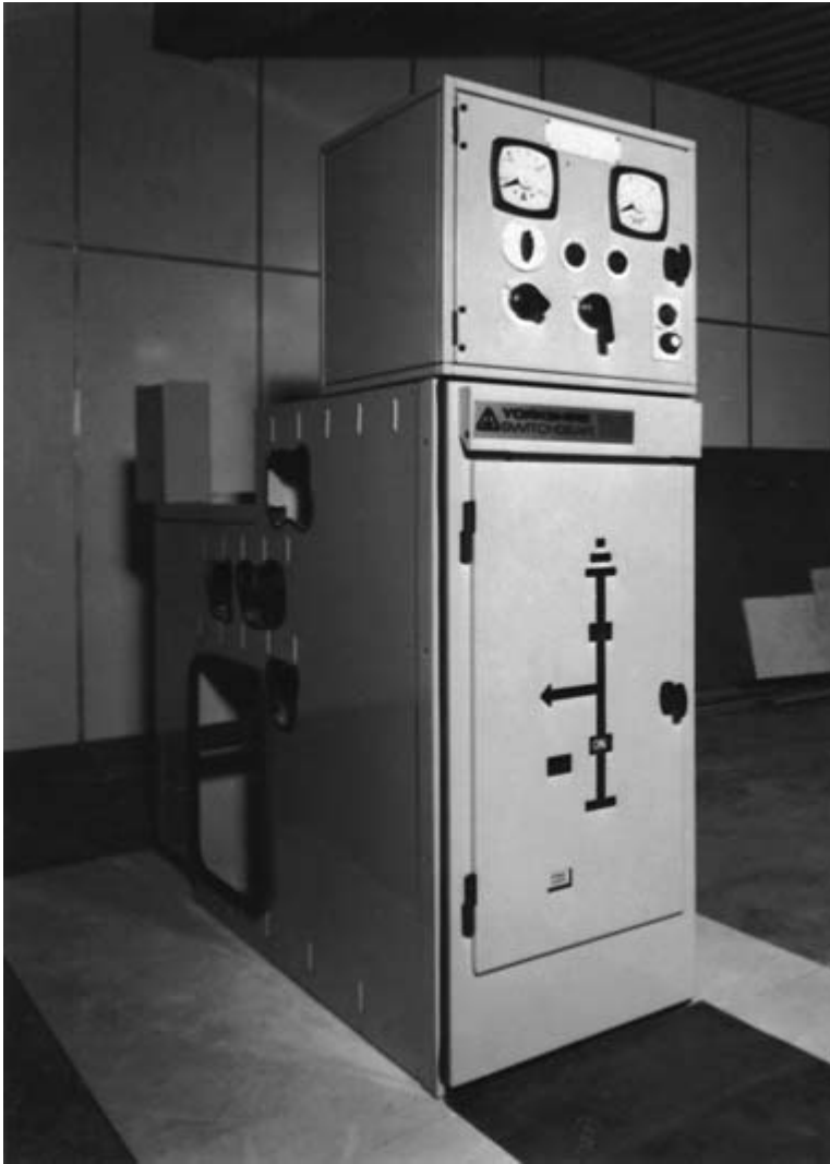
Fig. 14.11 SF 6 switchgear unit with horizontal withdrawal.
