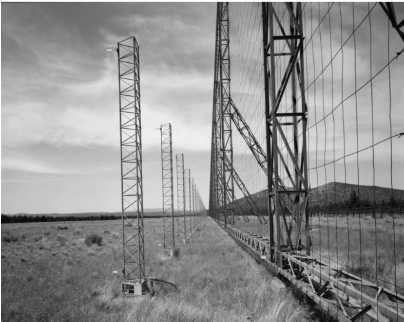
Figure 2.93 AN/FPS-18 radar: (a) the transmitter side and (b) the receiver side. (Source: Courtesy of Robert Hicks, NPS.)
