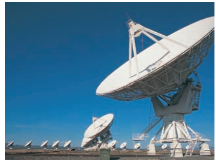
Telemetry receiving station for space satellites. © DV169/Getty Images RF
