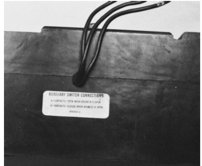
FIGURE 13-17 Auxiliary switch connection.
