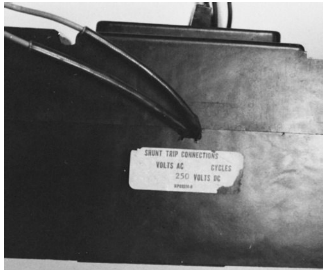
FIGURE 13-15 Shunt trip connection.
