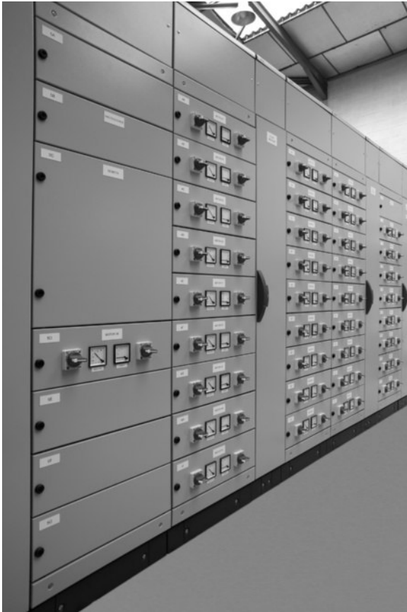
FIGURE 4-11 A typical power panelboard.
