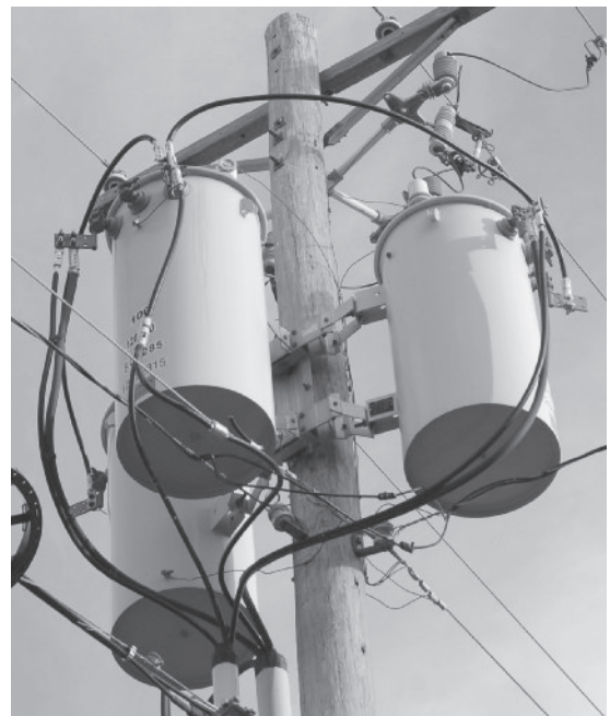
FIGURE 2-22 Single-phase transformers mounted on a pole and connected to form a 3-phase bank.
