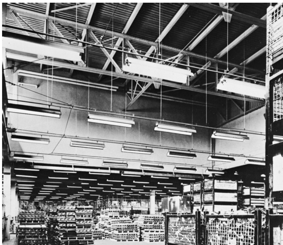
FIGURE 5-9 Typical trolley busway lighting system.
