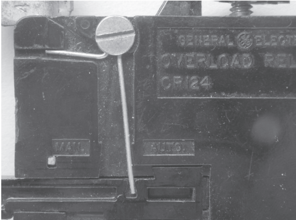
FIGURE 8-25 Bimetal strip overload relays can generally be set to permit automatic or manual reset of the auxiliary contacts.
