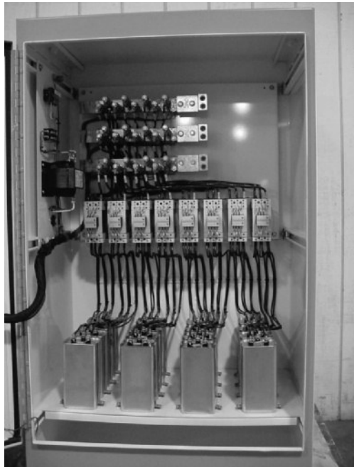
FIGURE 11-22 Capacitors used for power factor correction.
