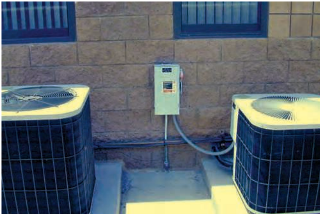
FIGURE 6-16 An application of liquidtight flexible metal conduit.
