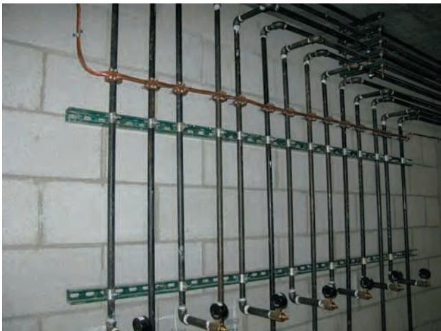
FIGURE 13-25 Bonding metal gas pipes.
