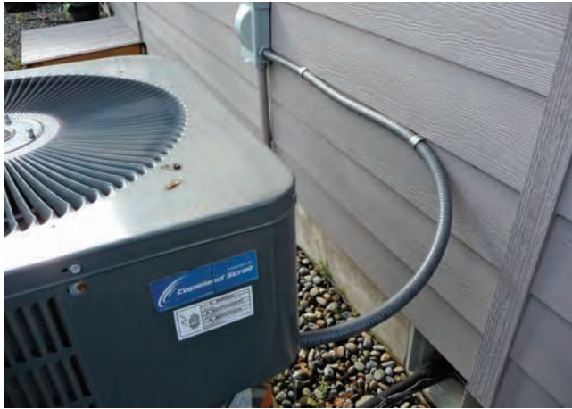
FIGURE 6-17 An application for liquidtight flexible nonmetallic conduit.
