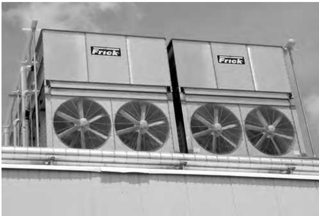
FIGURE 21-3 An evaporator with dual fans.
