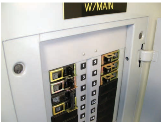
FIGURE 7-20 Circuit breaker–type lock-off accessory.
