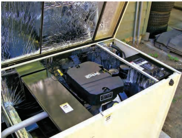
FIGURE 16-4 Generator suitable for emergency, legally required or standby power of the type generally specified for typical small commercial applications.
