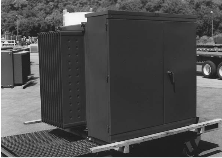
FIGURE 2.2.2 Typical three-phase pad-mounted distribution transformer. (By permission of ABB Inc., Jefferson City, MO.)
