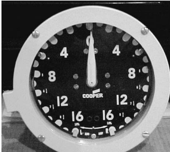
FIGURE 2.7.15 Tap-changer position indicator.
