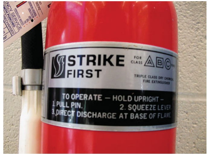
FIGURE 1-79 A typical fire extinguisher designed to be used on type A, B, or C fires.
