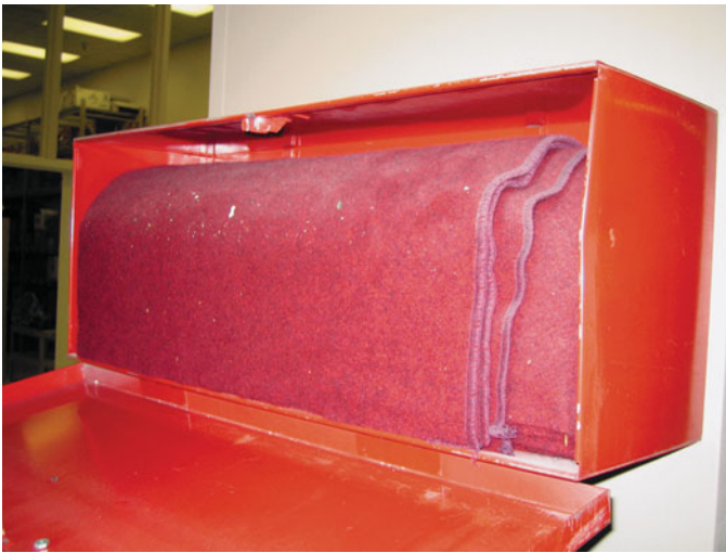
FIGURE 1-81 A treated wool blanket is kept in an easy-to-open, wall-mounted holder and should be placed in a central location in the shop.
