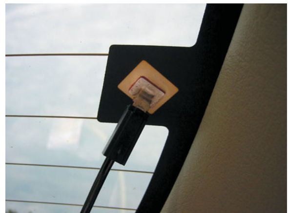
FIGURE 24-32 Corrosion or faults at the junction between the wiring and the rear window electrical grid are the source of many rear window defogger problems.
