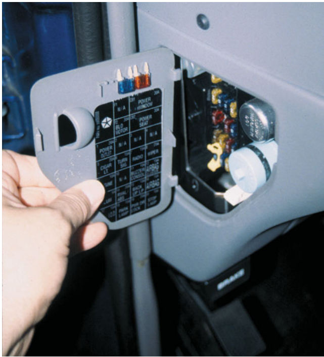
FIGURE 9-34 Always check the simple things first. Check the fuse for the circuit you are testing. Maybe a fault in another circuit controlled by the same fuse could have caused the fuse to blow. Use a test light to check that both sides of the fuse have voltage.
