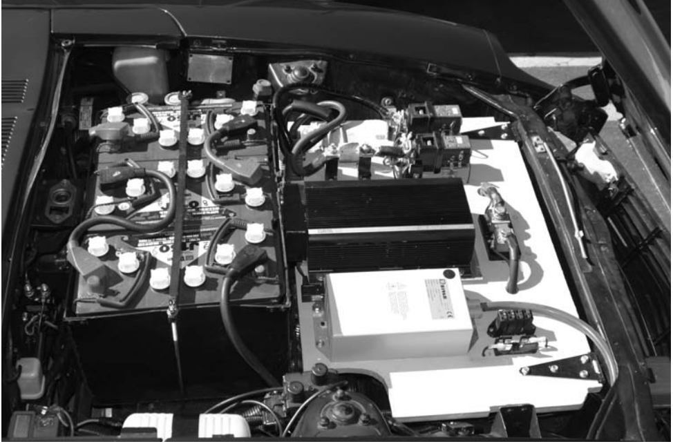
FIGURE 10-17 Operation Z battery mounted in place.
