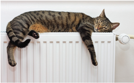
Figure 3.56 A room radiator.
