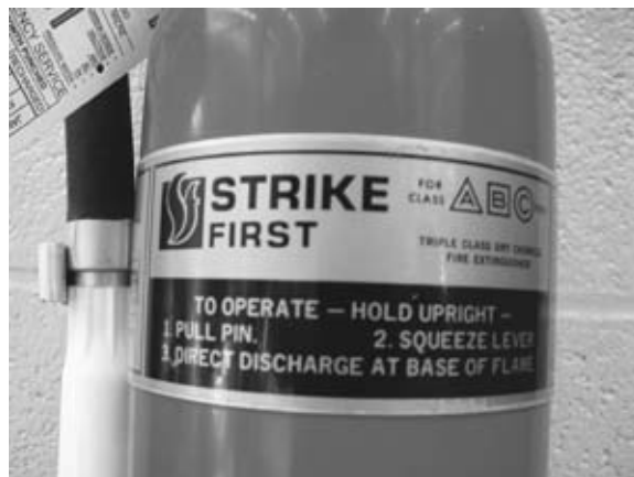
Figure 1-47. A typical fire extinguisher designed to be used on type A, B, or C fires.
