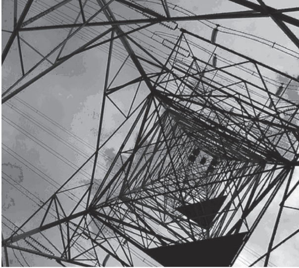
FIGURE 7.7 Steel lattice structure of a transmission line tower.
