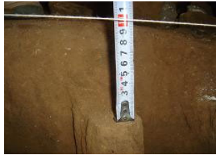
Fig. 11. The fracture position of fly ash-lime pile
