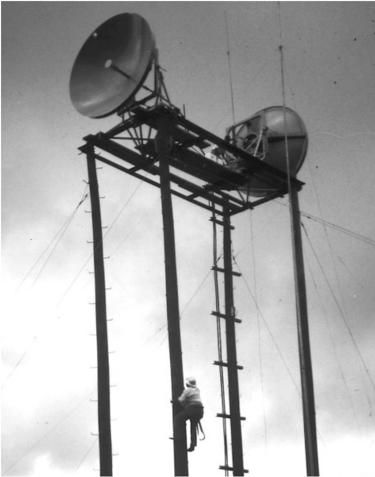
Figure 25.14 Provisional radio-relay tower in Guatemala, 1968. (Courtesy of Gerd Lupke.)
