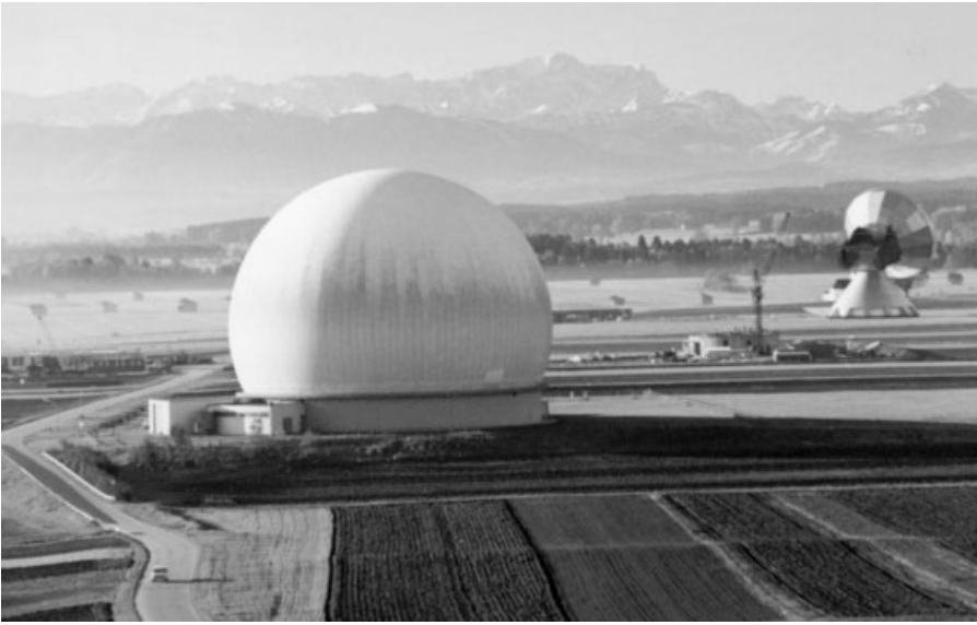
Figure 27.4 Earth station at Raisting, Germany. (Courtesy of Museum für Kommunikation, Frankfurt, Germany.)
