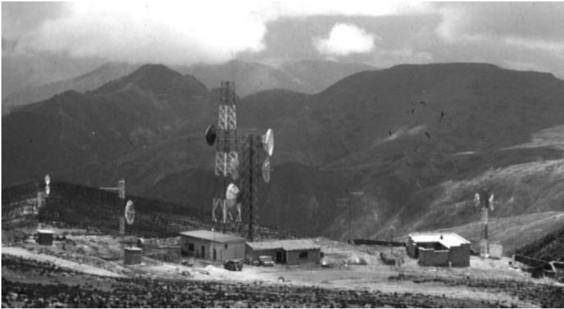
Figure 25.7 World's second-highest broadband radio-relay repeater, in Bolivia. (Courtesy of Siemens.)
