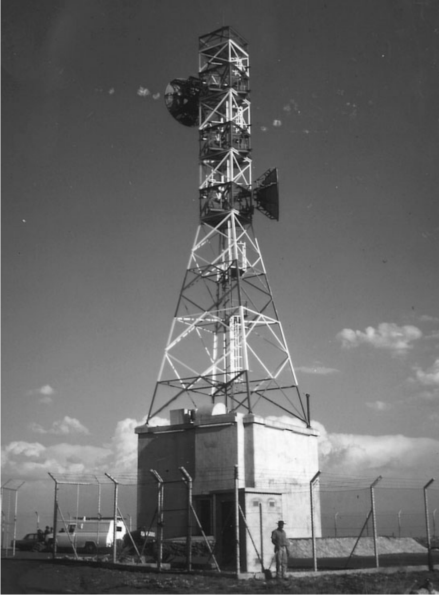
Figure 25.11 Radio-relay repeater station in South Africa. (Courtesy of Gerd Lupke.)
