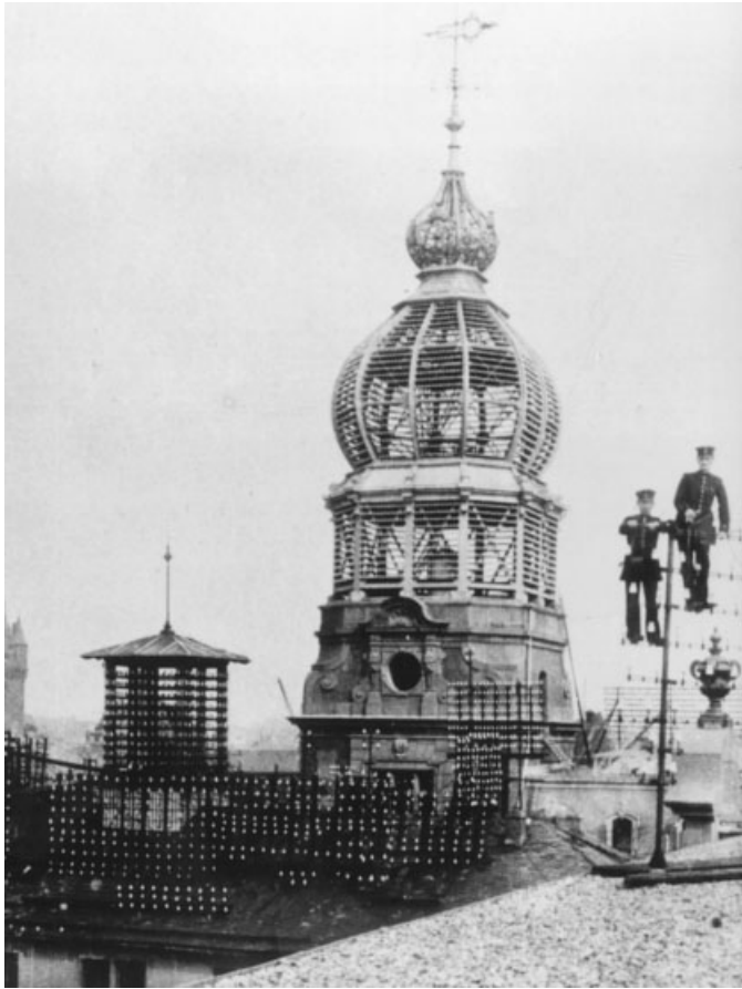
Figure 20.2 Open-wire support and access tower on the roof of a telephone exchange. (Courtesy of Museum für Kommunikation, Frankfurt, Germany.)
