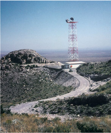
Figure 25.1 Typical radio-relay repeater station in Thailand. (Courtesy of Gerd Lupke.)
