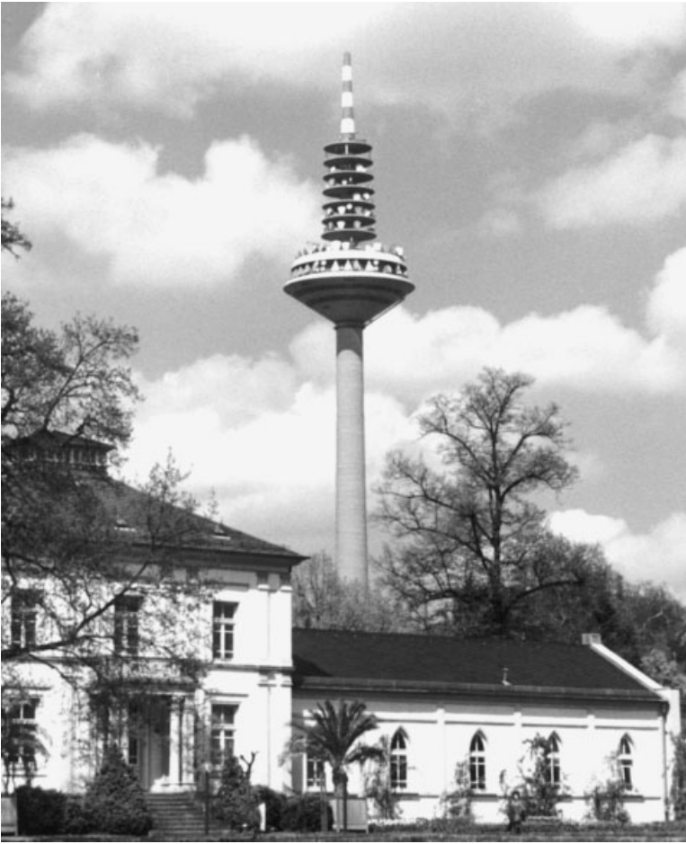
Figure 25.19 Highest telecommunications tower in Germany, at Frankfurt, with the world's largest antenna platform.
