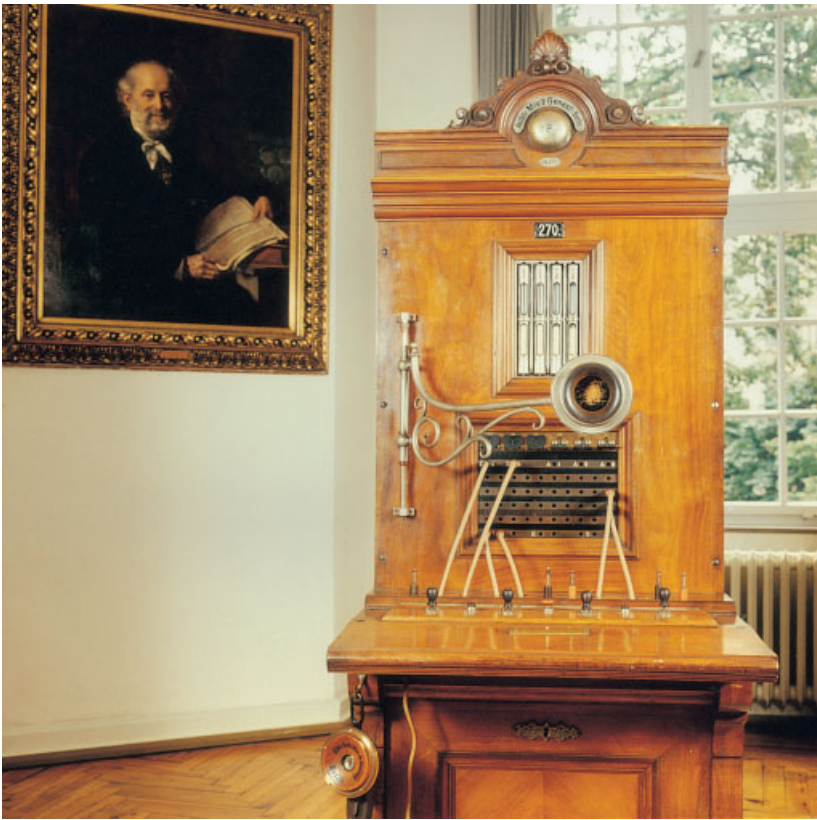
Figure 11.3 Manual exchange used in Germany around 1900. (Courtesy of Alcatel SEL.)
