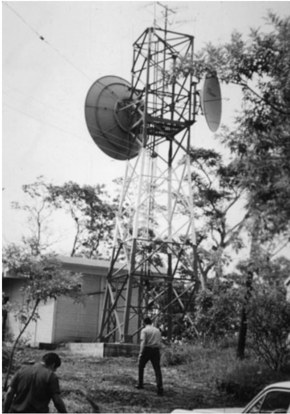
Figure 25.6 Typical radio-relay repeater station in Central America: the Las Pavas station in El Salvador, 1968.
