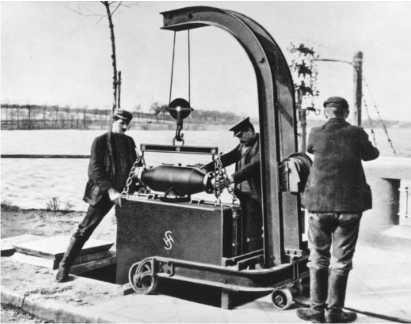
Figure 20.8 Placing of a Pupin coil in a cable duct, 1912. (Courtesy of Museum für Kommunikation, Frankfurt, Germany.)
