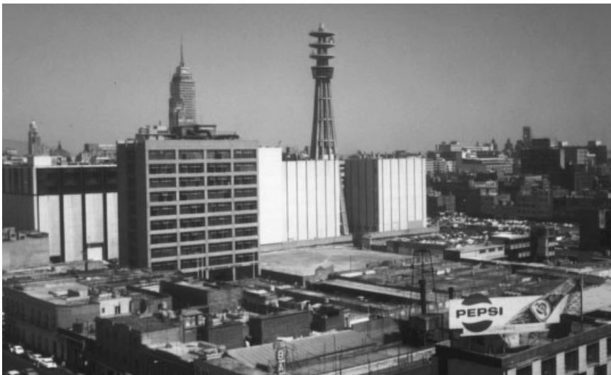
Figure 25.18 Telmex radio-relay tower in Mexico City, 1960. (Courtesy of Gerd Lupke.)
