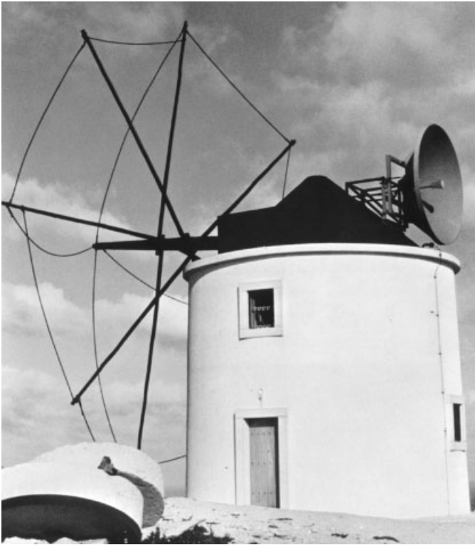
Figure 25.16 Ancient windmill used as radio-relay station at Sesimbra, Portugal, 1973. (Courtesy of Alcatel SEL.)
