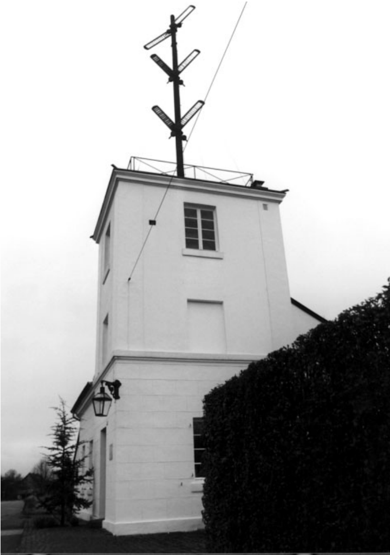
Figure 5.5 Restored optical telegraph station at Cologne. (Courtesy of Museum Optischer Telegraph, Köln-Flittard, Germany.)
