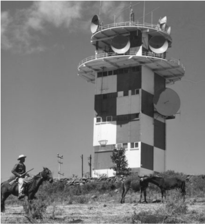
Figure 25.5 Radio-relay repeater station on Mount Culiacan, Mexico. (Courtesy of Alcatel SEL.)
