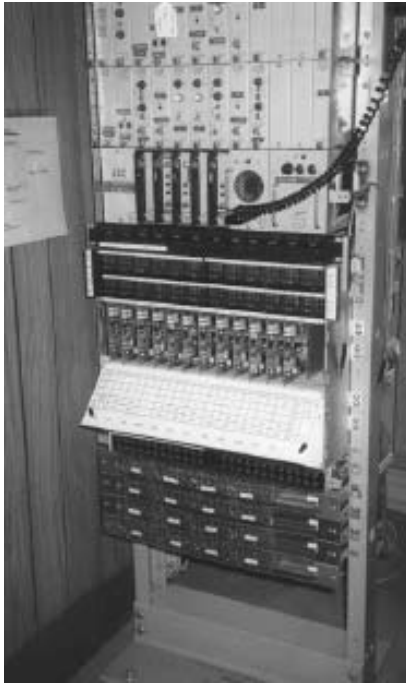
Figure 3: A 12-channel frequency division multiplexing (FDM) equipment bank used in an analog microwave system for telephony. Copyright © 2002 Dave Whitmore. Reprinted by permission.
