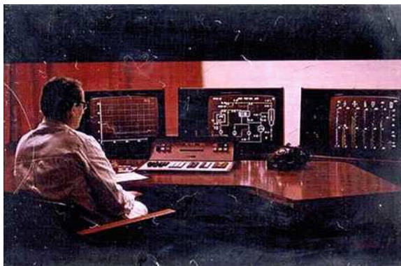
Fig. 2.1 The OPCOM control room
