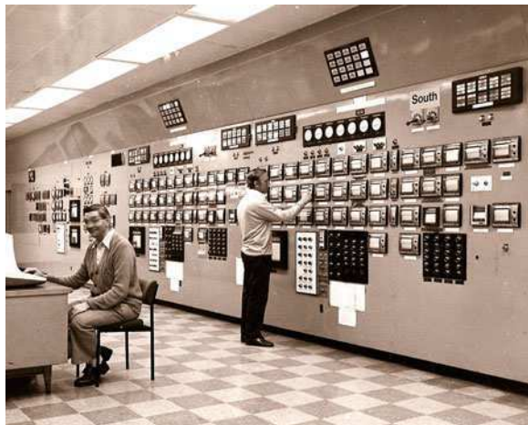
Fig. 8.1 A typical conventional panel from a process plant operating in the 80s
