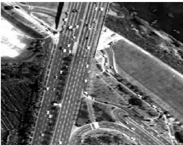
Fig. 4 Google Earth view of a unregulated intersection
