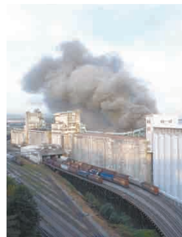
Figure 6.8 Mixtures of grain or coal dust and air are potentially explosive, as shown in this grain elevator explosion.
