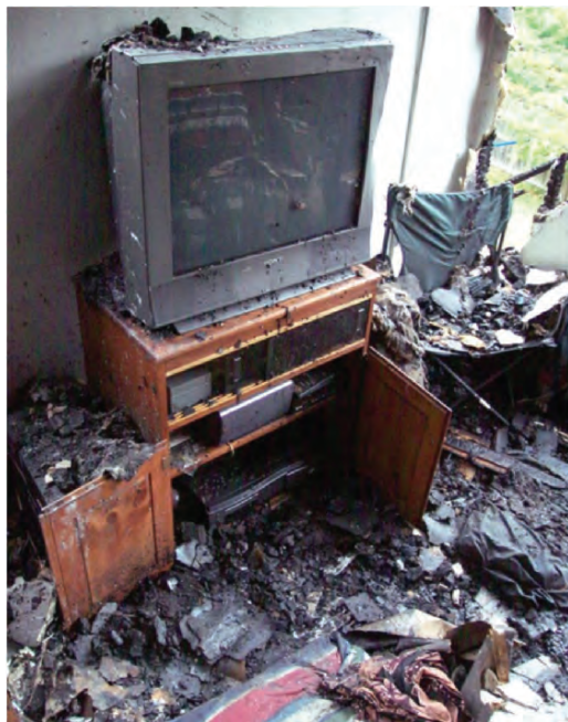
Figure 5.42. Photograph of damage from a candle-ignited fire that destroyed a campus fraternity house in Amherst, MA. Flame retardants likely prevented the television and surface-treated wood cabinet from igniting. Reproduced from http://www.buildinggreen.com .
