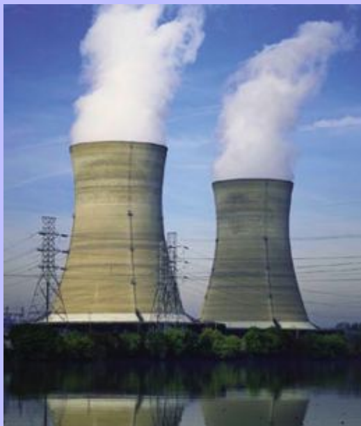
Power plants require large cooling towers to dissipate heat.
