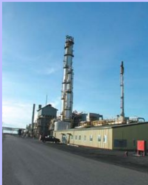
Ammonia for fertilizer is produced in reaction towers at elevated temperature and pressure.
