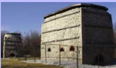
Older limestone kilns have air vents through which \text{CO}_2 can escape.
